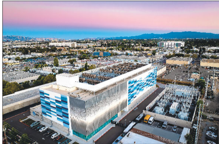
A LARGE NTT data center rises in a Santa Clara neighborhood. An association of locally run electricity providers has called on state officials to analyze how quickly demand is increasing.
